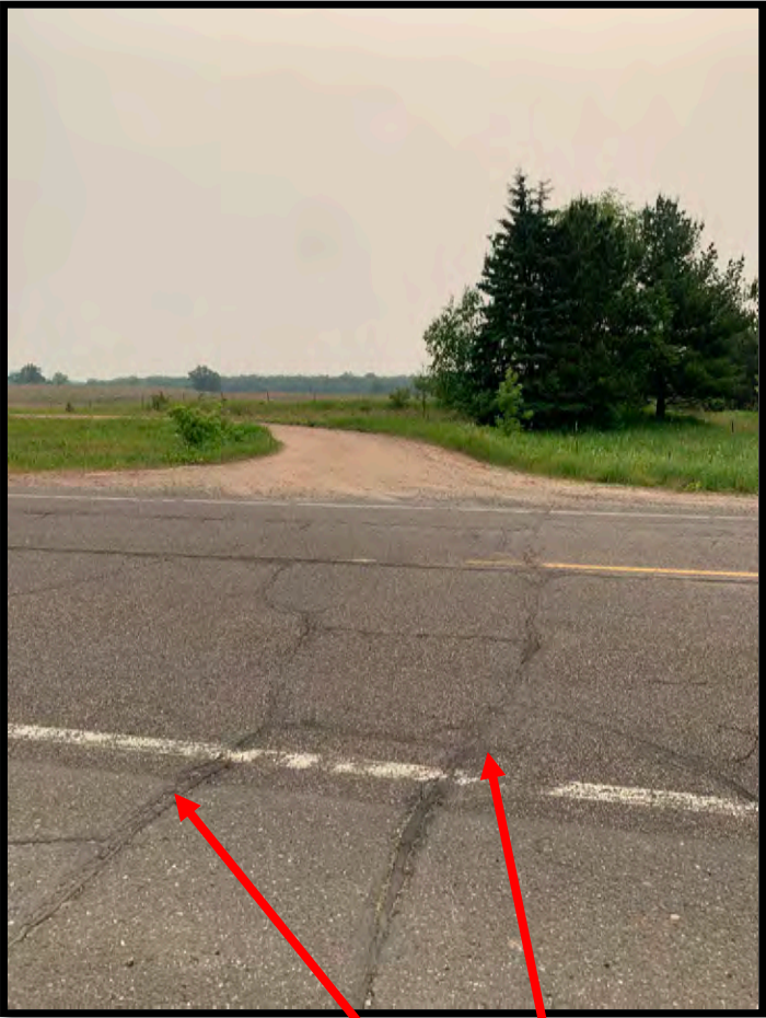
Transverse cracking
